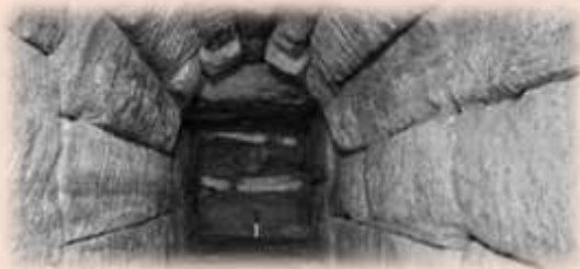
Church Street sewer, York
